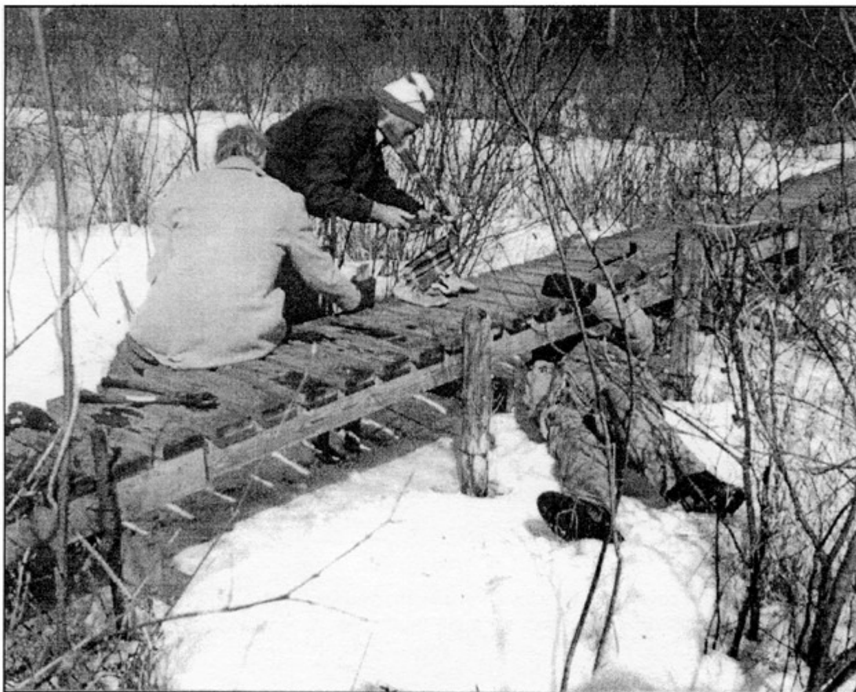
Maintenance work on the Marion Webb bridge in the Gould Lake Conservation Area.
