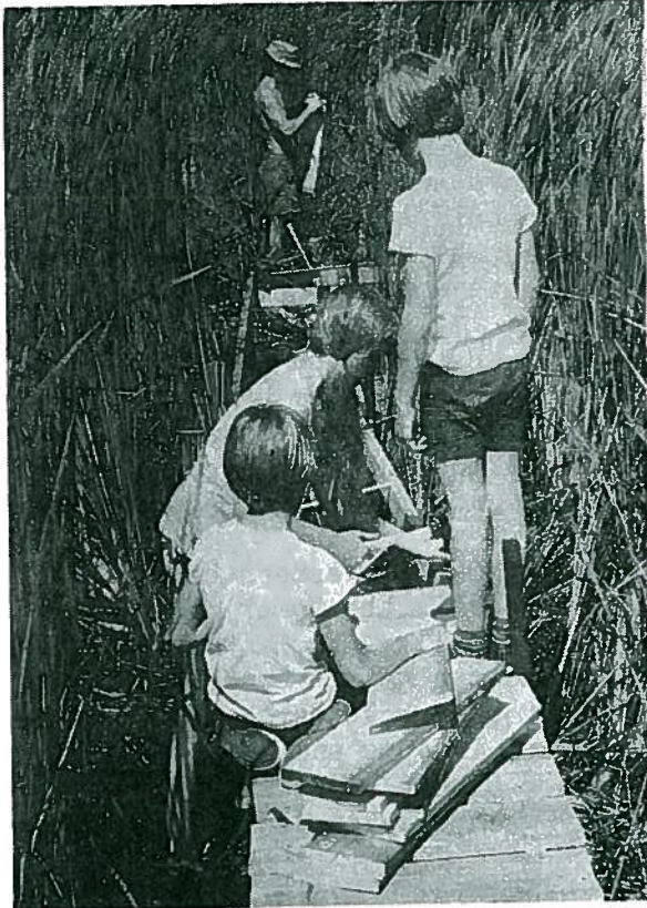
Building the catwalk Four-sixths of Doug Knapp's family
