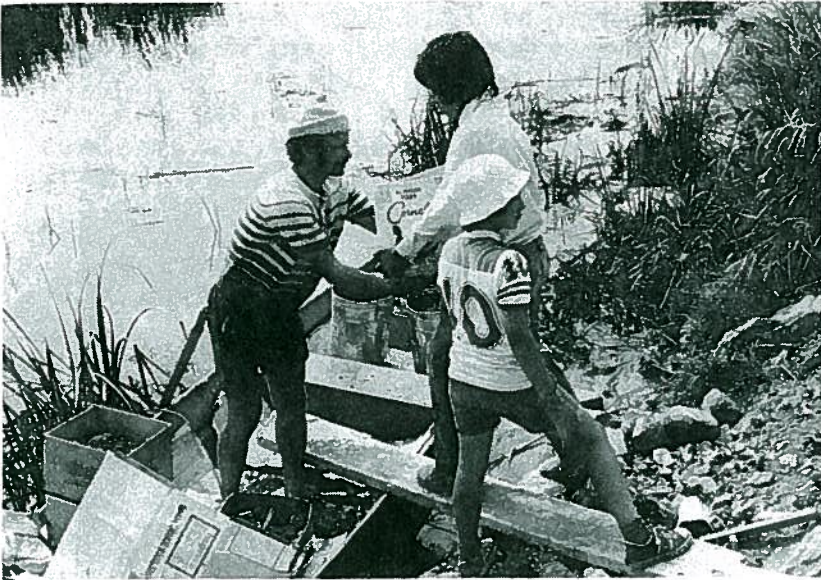
Loading the rock for the gabions Oh my aching back!
