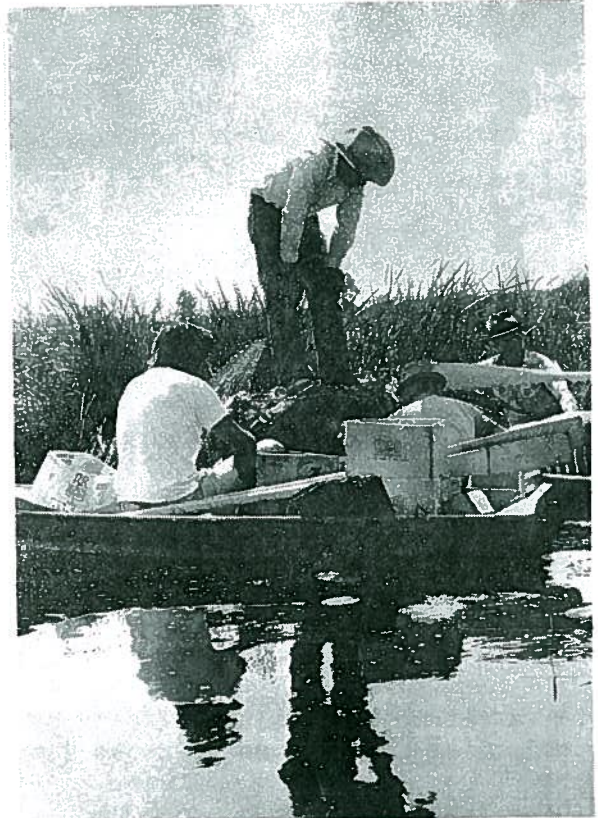
Filling the bridge gabions Bill Cotton (foreman) cracking the whip
