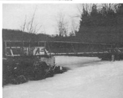
Right: the completed bridge.
