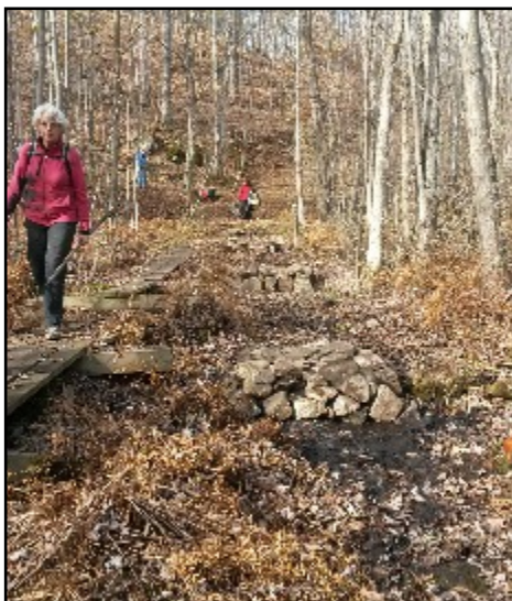
Stone piers instead of wood footings Right: Section construction in CRCA workshop.
