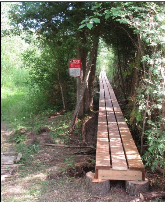
Boardwalk construction near Ottawa's Paden Rd. Is well underway. STEVE KELLY
