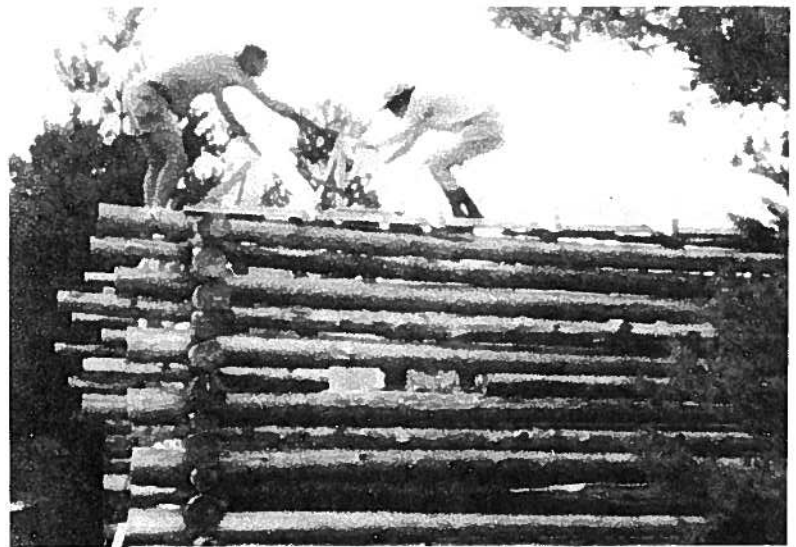
(Left) Summer, 1978. The trusses are up and the work party is ready to go home. Chinking between the logs and cutting out the door and windows were the next jobs.
