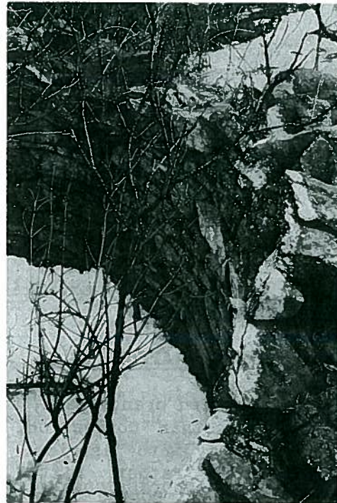
The wall of the lime kiln on the trail near Gilroy Road. Photo by Don Mitchell.
