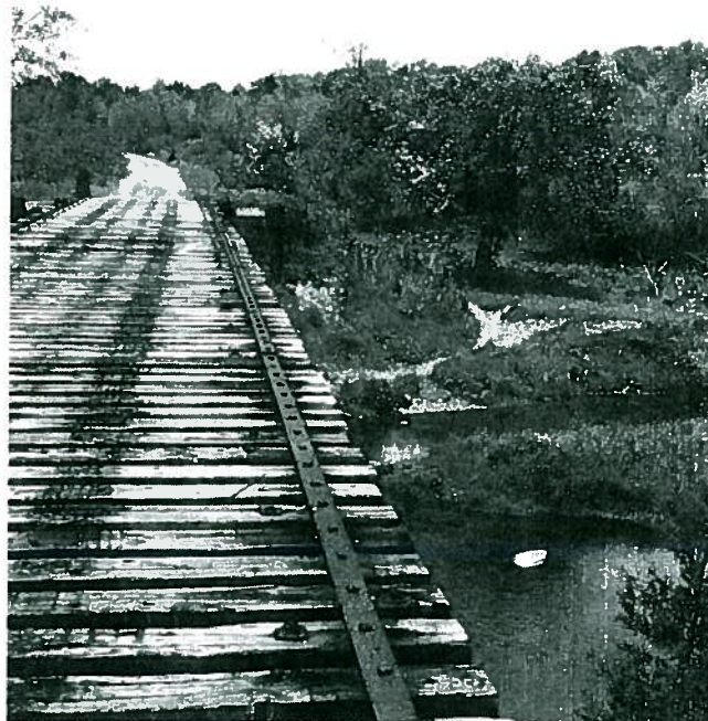
Lynn Valley Trail Bridge
