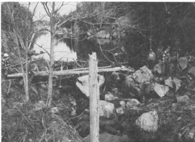
"Devil's Gorge" bridge under construction
